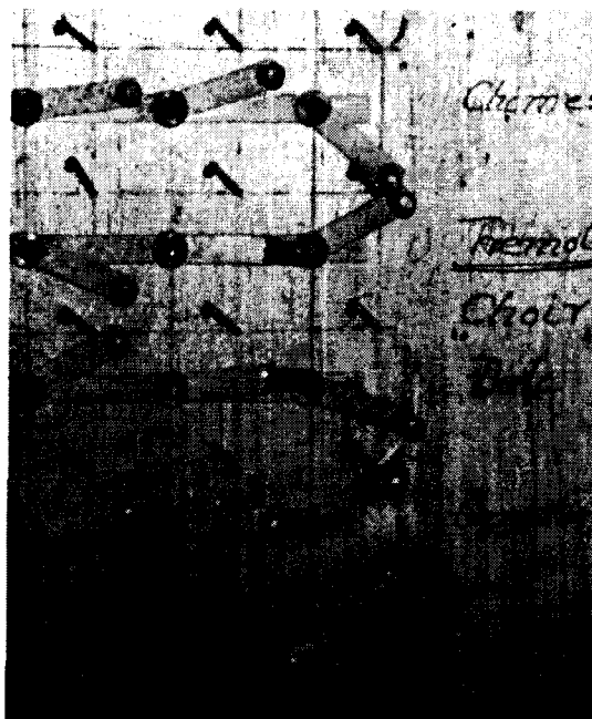
A close-up look at the factory switching panel
