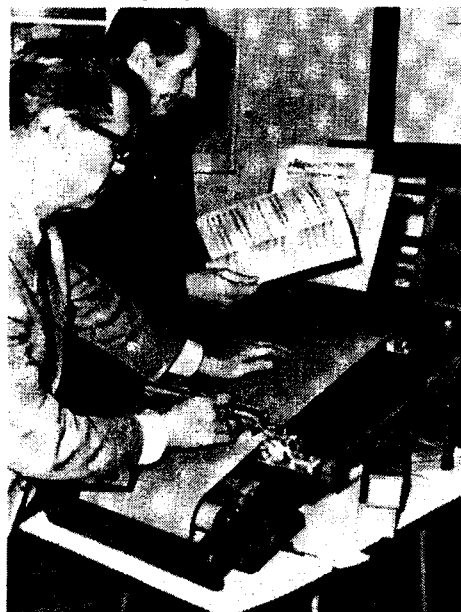
Victor Zuck (foreground) registering a roll on the portable registering punch.
